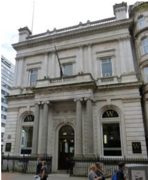
Figure 1 - Midland Bank, corner of New Street and Stephenson Street, Birmingham
