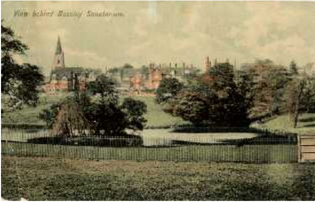
Left: The view across Moseley park and pool to Chantry Road and St Anne's church
