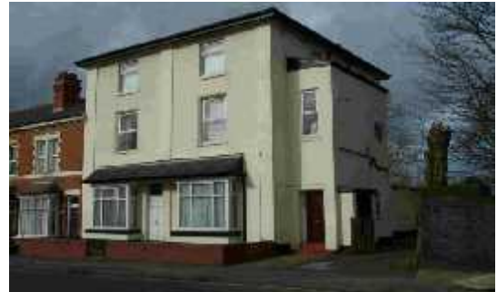
Below: Building damaged by World War II bomb
