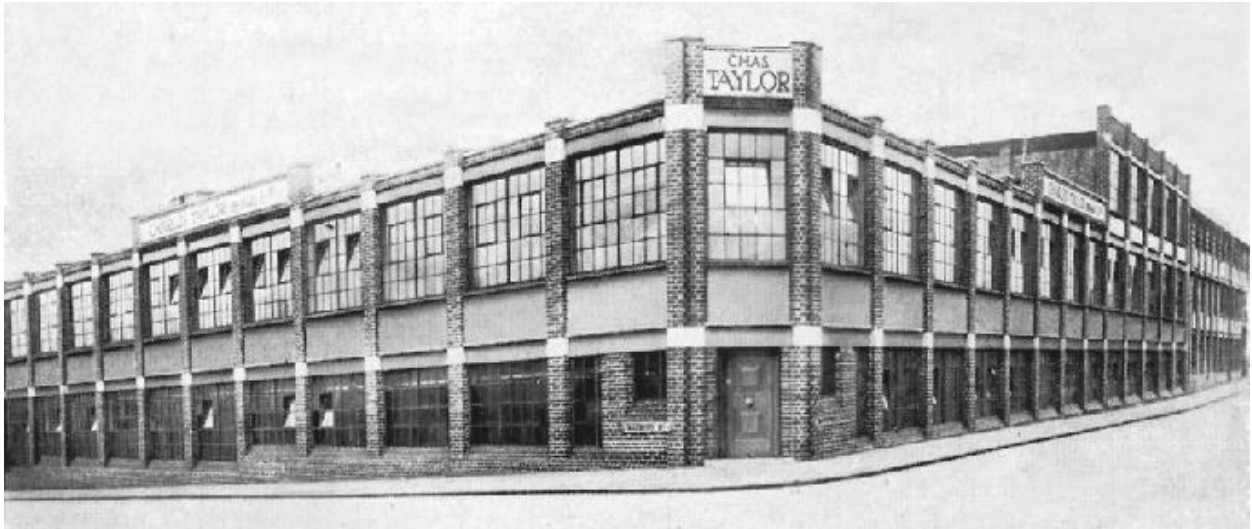
Figure 7: Charles Taylor works in Bartholomew Street, Birmingham
