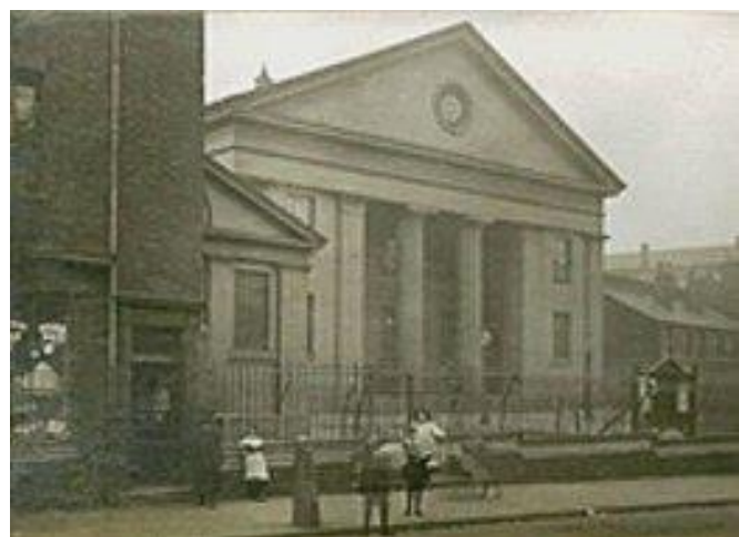
Figure 3 The Non-Conformist Church of the Saviour in Edward Street, Birmingham
